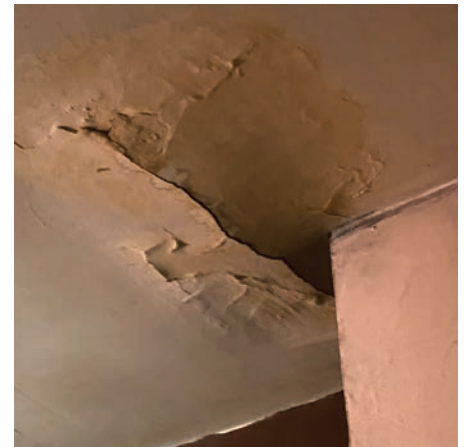
Damage caused by leaking roof
